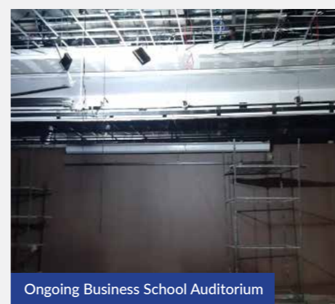
Ongoing Business School Auditorium
