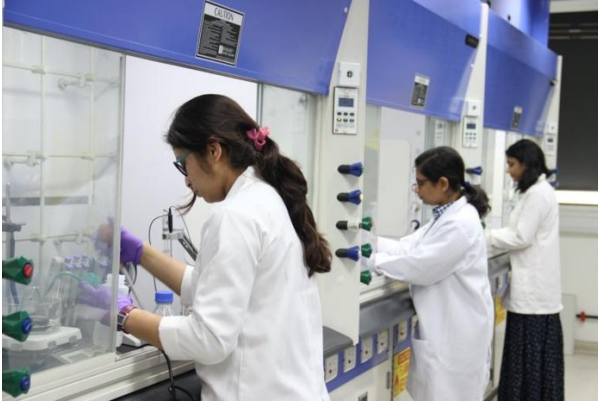
Wet Lab Fume Hoods for chemical work
