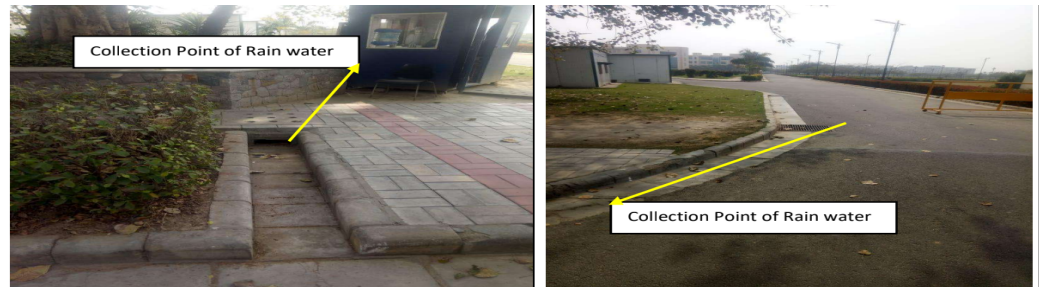
Figure 6 Stormwater drainage and catchment
