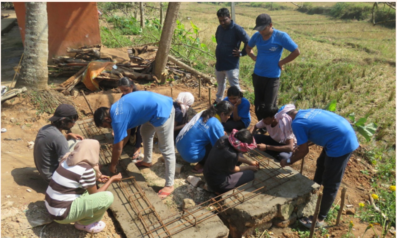
Our second batch students helping with the construction of an individual toilet-cum-bathroom in Tuburuda Village, Gajapati District during their field education course with Gram Vikas, Odisha
