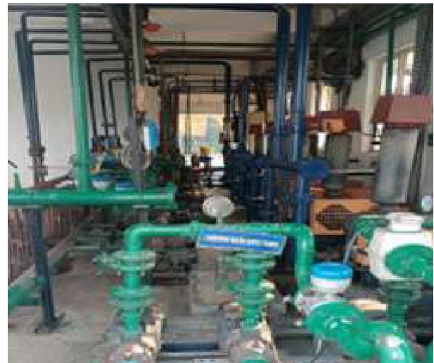
Gardening water supply pumps for reuse of treated water
