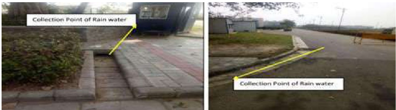
Stormwater drainage and catchment
