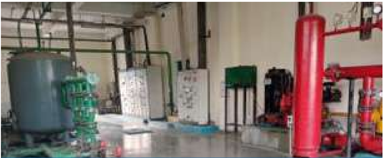
Water Treatment Plant
