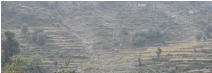
Land Erosion in Ukhimath causing land to 'sink' and 'slide'. These particular scars were formed during the 2013 disaster in Uttarakhand.
