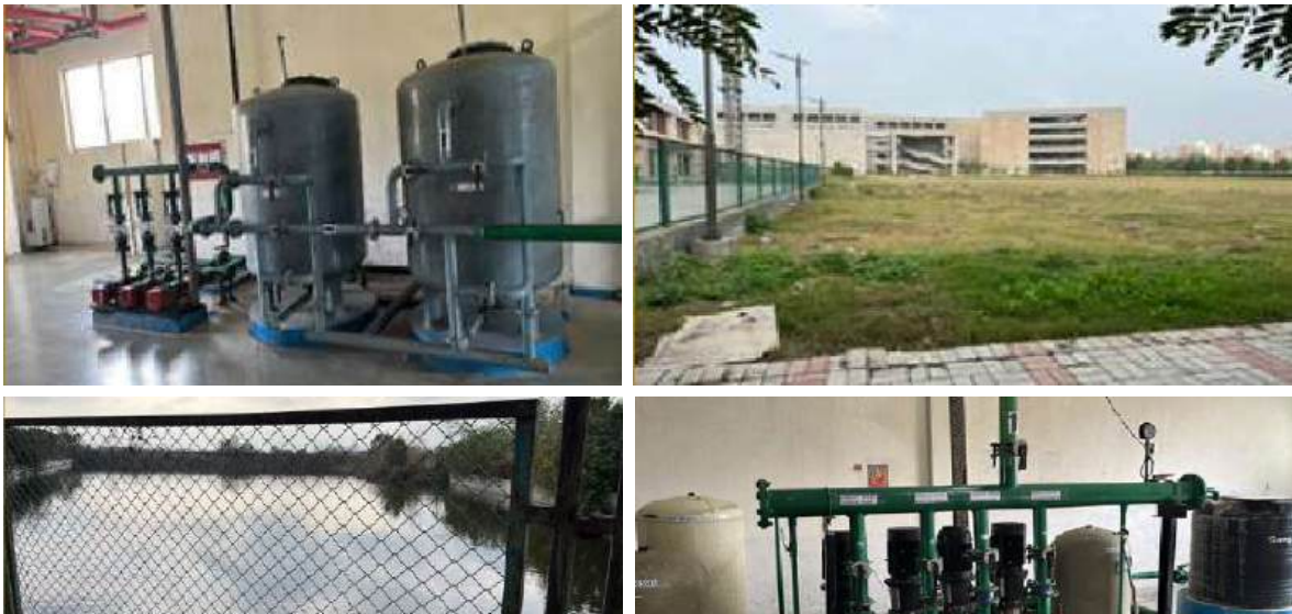
STP 150 KLD: This modular-type plant (50+100) treats water from campus
