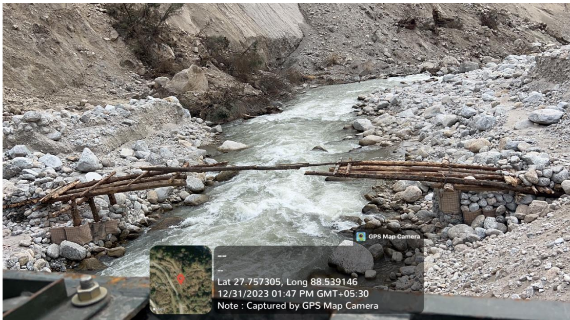
Picture 5. Log bridges constructed by the Dzumsa for the movement of livestock 6
