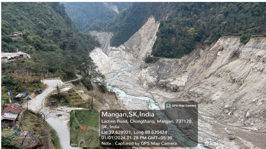
Picture 2. Daray Village on the right bank completely washed away
